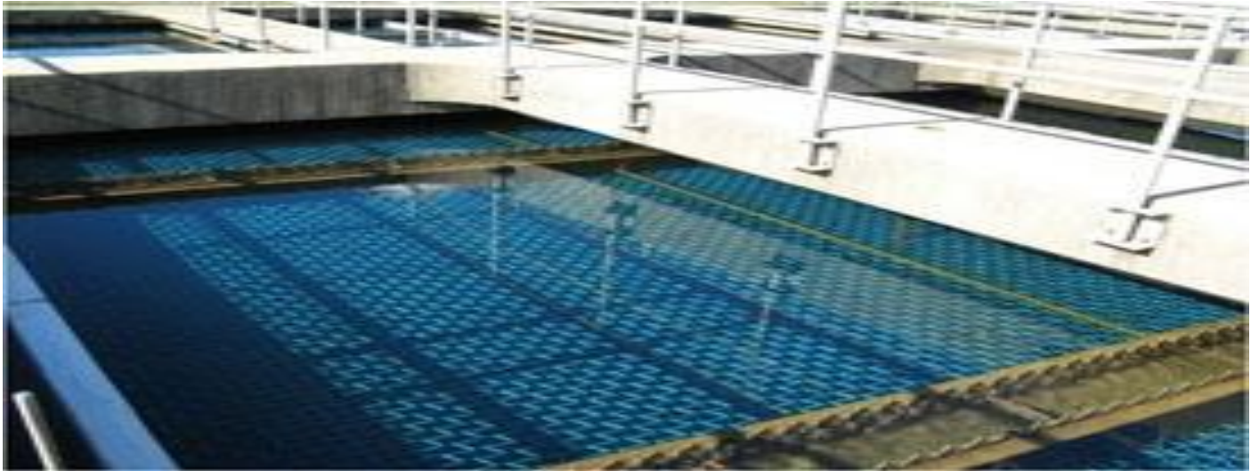
Lexington Water Treatment Plant Basins
