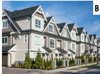
Parking in rear with gable roof
