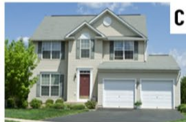
Two-story with front garage
