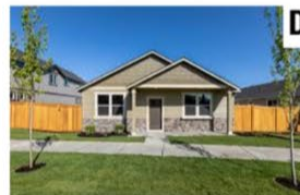
One-story with no garage
