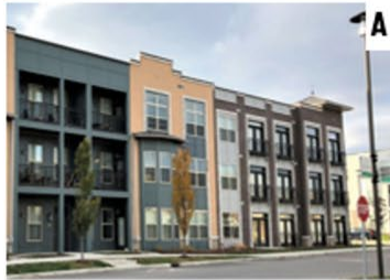
Parking in rear with flat roof
